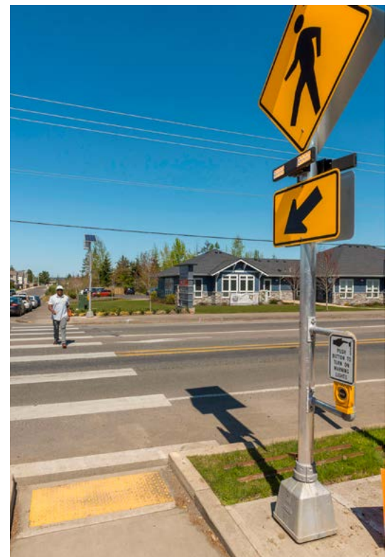
Example of a completed Rectangular Rapid Flashing Beacon (RRFB) crossing, creating a safer and more visible pedestrian crossing along a busy corridor.
